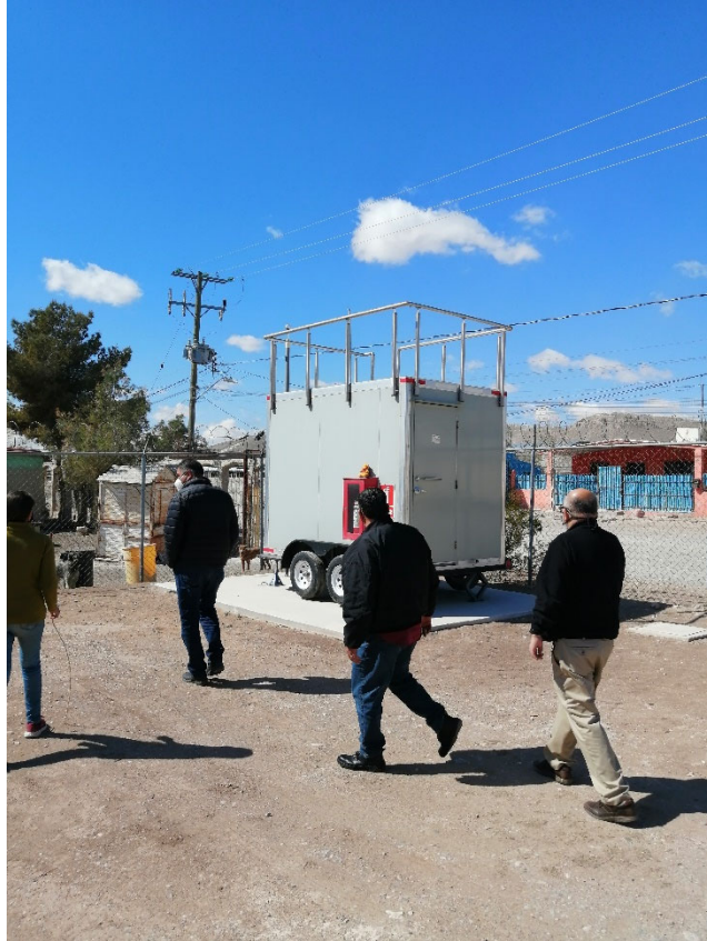
Picture 15 – Monitoring Equipment at site
